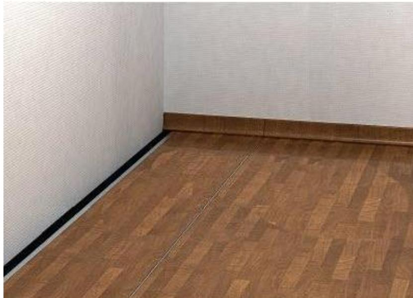
Then cover the area towards the room with the appropriate floor material. The covers are fixed in the aluminium profile in the locking brackets and the joints are supported by joint seals (3 pieces at 2 m).
