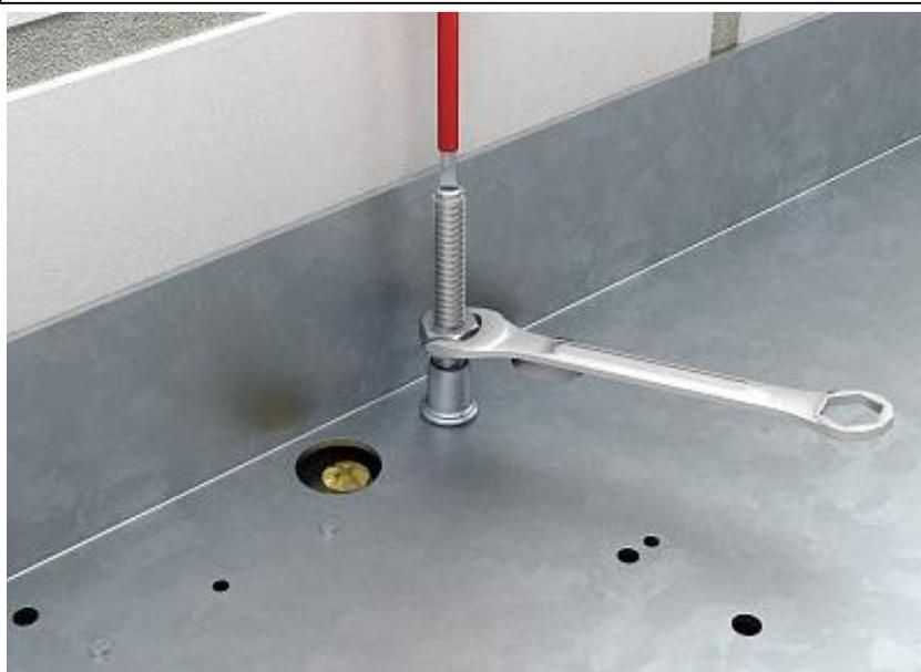
Fine adjust the trunking units to the top edge of the screed. Fasten the floor plates of the levelling unit on the raw ceiling. Check the height adjustment of the height-adjustment units and secure using a locknut.
